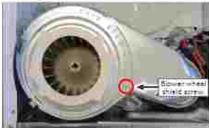
Figure 2 - Blower wheel shield screw
