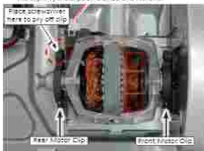
Figure 4 - Drive motor retaining clips
