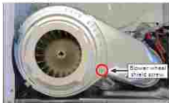
Figure 2 - Blower wheel shield screw
